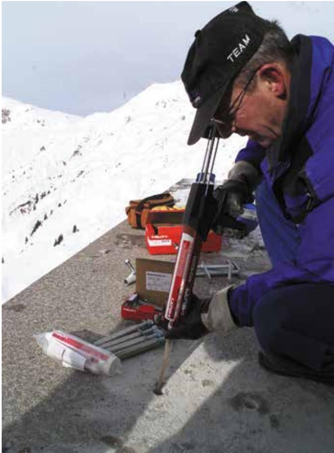
**Fig. 2: Injecting adhesive using a hand-operated injection tool—the adhesive is mixed in the static mixer attached to the end of the tool. The MPII must be consulted to ensure that the adhesive is appropriate for the ambient conditions**
